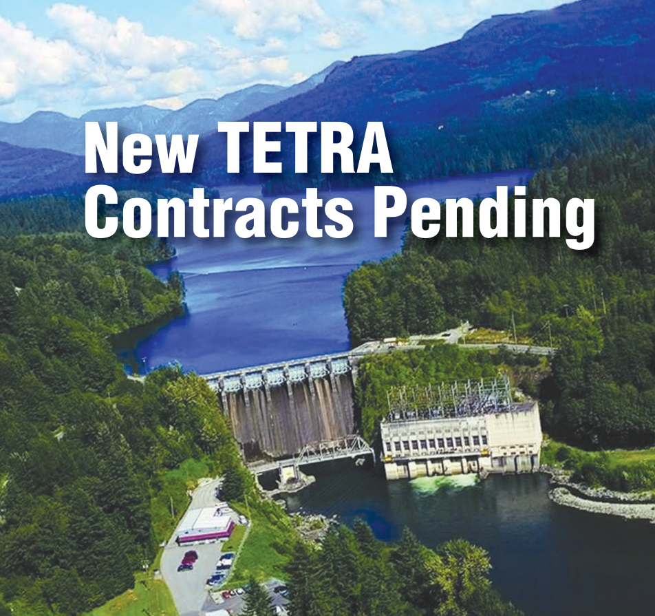
Photo courtesy BC Hydro
